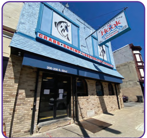
Photo by Daria Williams | Mr. Hook storefront after renovation
